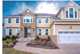
17-03 Gates Place, Wayne
